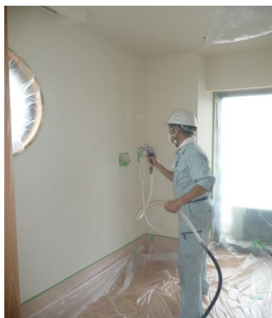
【 Applied 'LUMITITAN-NAG' with spray gun (Vertical) 】
