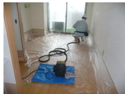
【 Applied 'LUMITITAN-NAG' with spray gun (Horizontal) 】
