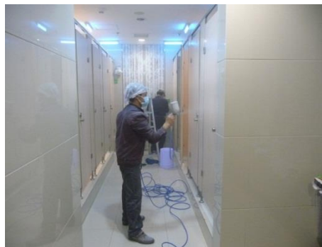
Applied to restroom doors
