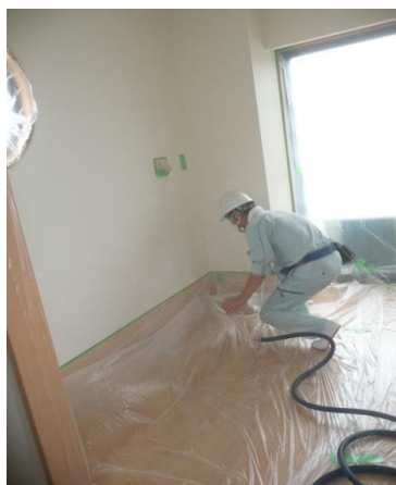
【 Applied 'LUMITITAN-NAG' with spray gun (Vertical) 】
