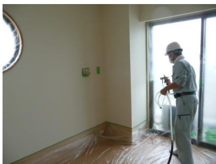
【 Applied 'LUMITITAN-NAG' with spray gun (Horizontal) 】
